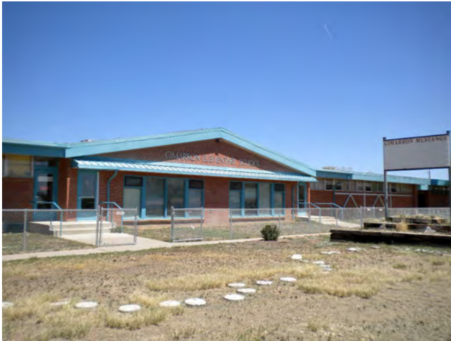
Elementary school wing (1965 orig.)
